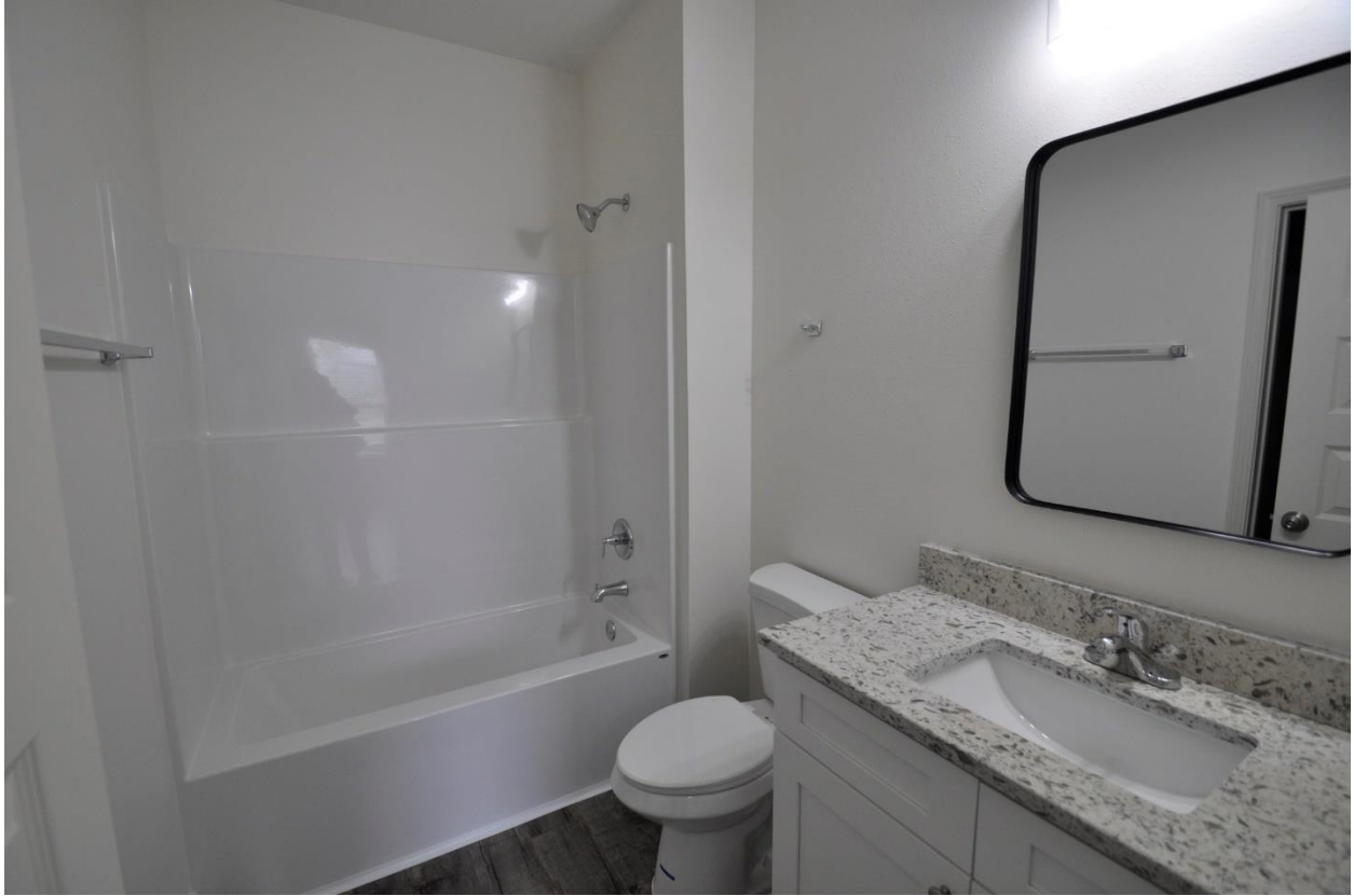
Primary Bathroom of unit B
